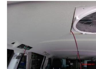
36 Inside, the wires are fed through the hole in the spacer across to the c pillar
