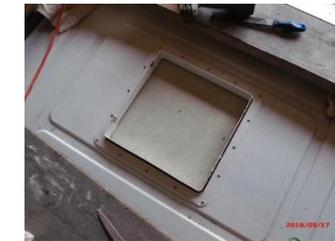
33 Sealant is applied and all screws secured.
