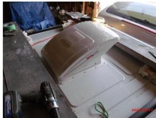
35 With the fan open, 4 screws attach it to the mount (it was checked for operation before cutting the hole)
