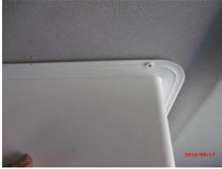
25 the final position of the inside frame can be set to avoid the ridge in the liner
