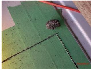
29 so none of the metal dust would fall into the van and could be picked up with a magnet
