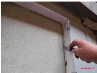
34 The liner cuts easily with a serrated knife. Note the hole in the wood spacer for the wires.
