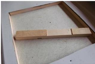
31 A 3/4" pine spacer between the roof and liner gives enough depth to mount the fan and something to screw into. Notches provide room for the sound proofing and wires
